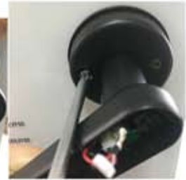
4. Put front handle onto door and get the rod through hole on lock body
